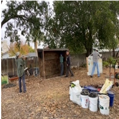
The old shed emptied and the start of the demolition.
