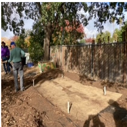
This is where the new shed will go.
