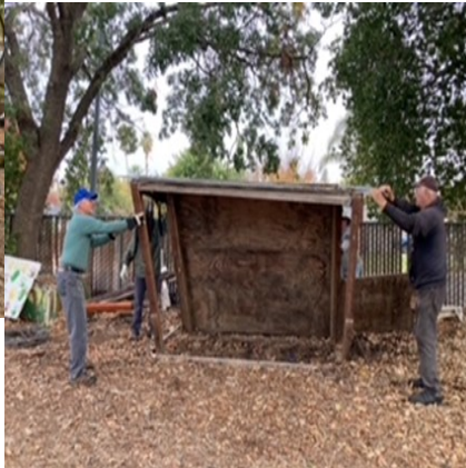
Old shed about to come down.
